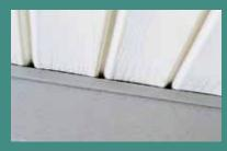
DRDINARY SOFFIT LACKS STIFFNESS, SO IT ENDS TO CUP WHEN INSTALLED.
